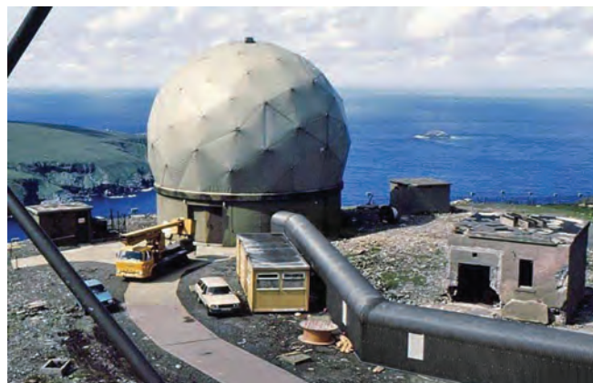
HF200 radar beneath the radome and covered walkway to the R10 operations block on the hillside below
